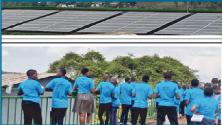
Students observing solar panel installation
